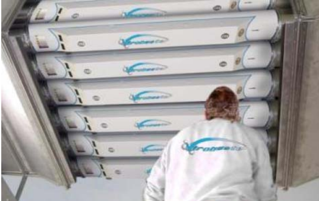
Fig 4.2 Installation of Virobuster Steritubes in Plenum Ductwork
